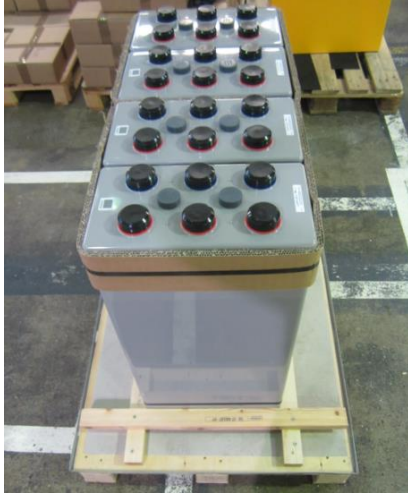
Battery cells are positioned and fixed with wooden beams on an EUR-pallet, strapped on top with cardboard in between.
