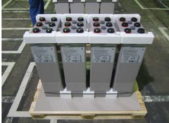
Battery cells are positioned with polystyrene forms on an EUR-pallet and strapped on top.
